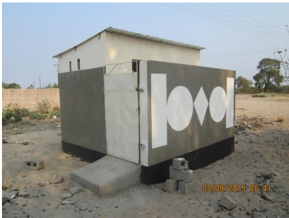
Front and back of the VIP (ventilation improved pit latrine).
