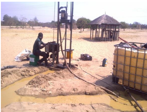
Construction of the new borehole.
