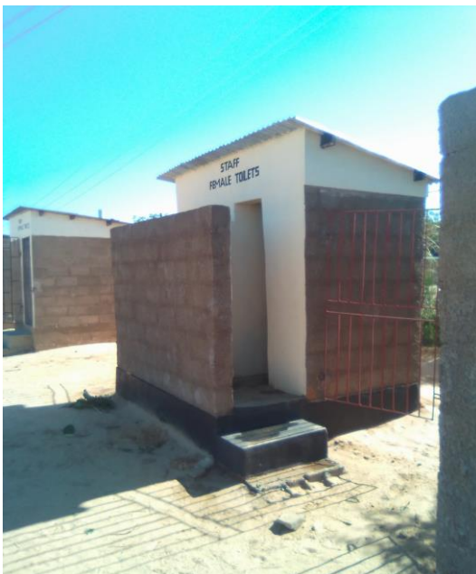
Toilets for staff
