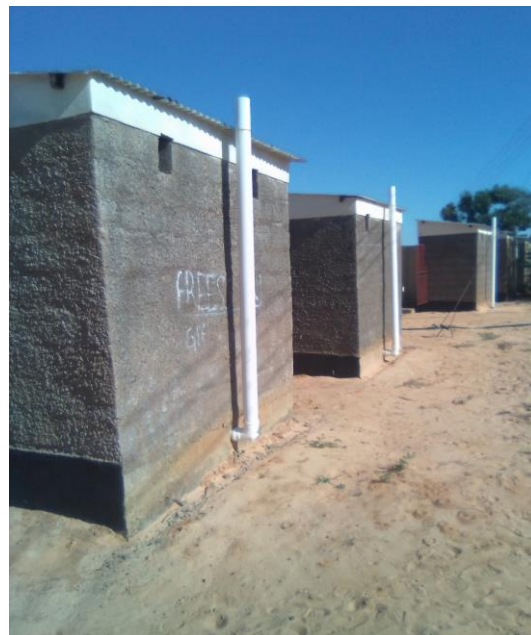
Back of the toilets
